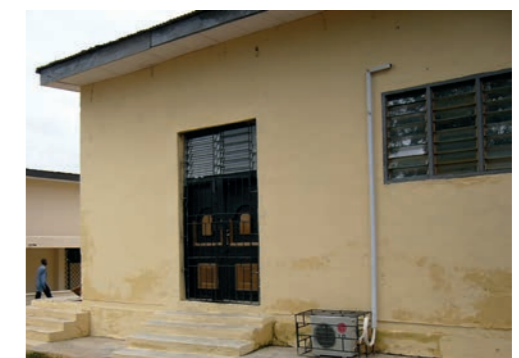
Secure storeroom with windows to ensure adequate ventilation, Nigeria
